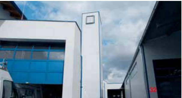
Because of the surrounding vehicle infrastructure, the LogiMat was constructed against the outer facade of the warehouse and outfitted with panelling.
